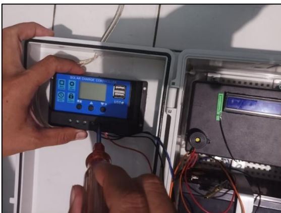
Gambar 8. Memasang solar charge controller.
