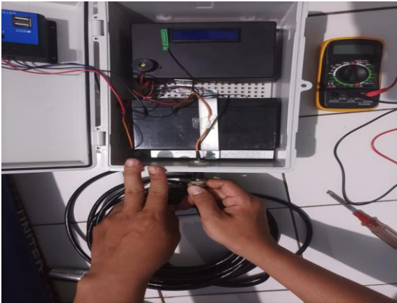
Gambar 11. Memasang kabel sensor pressure.
